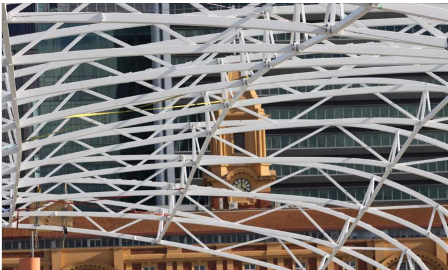
In front of the landmark Ferry Building is stunning steelwork fabricated in Napier.
