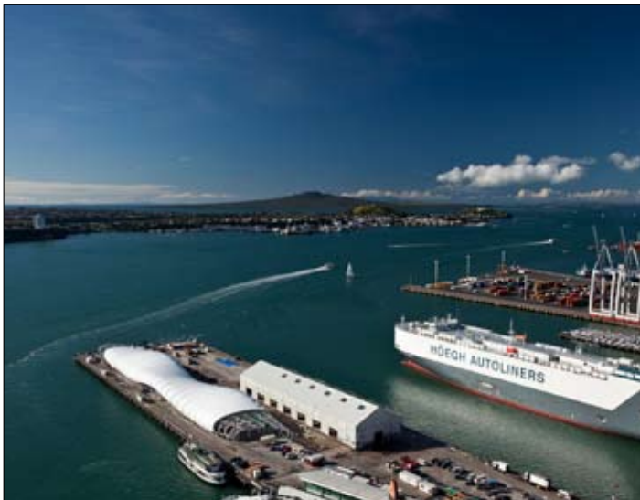
Beside Shed 10, The Cloud is clad in PVC and will have transparent walls of ETFE.
